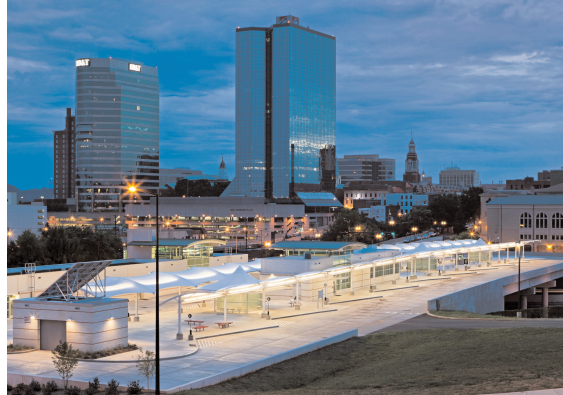
CDM Smith won The Grand Iris Award, the highest honor in the 2012 EEA competition, for its project, John J. Duncan, Jr. Knoxville Station Transit Center. The Transit Center is owned by the City of Knoxville and operated by Knoxville Area Transit. Entries for the 2013 EEA competition must be submitted by November 2.
